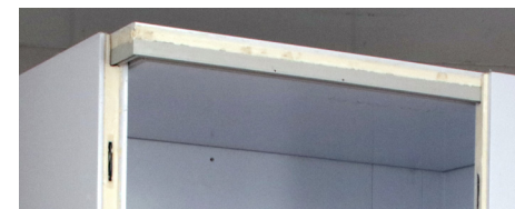
PARTICOLARE INCASTRO | PANELS JOINT
